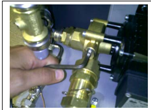
Figure 7 – Priming Screw on Pump
