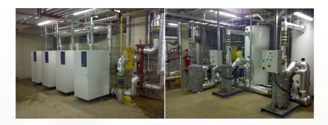
Gas-fired boilers, system seperation plate heat exchangers, HWS plate heat exchangers and HWS buffer vessels from MHG Heating are helping Berkeley First to keep the post graduates of Imperial College warm and clean at the 500+ bed accommodation blocks recentley built in Clapham, South West London.
